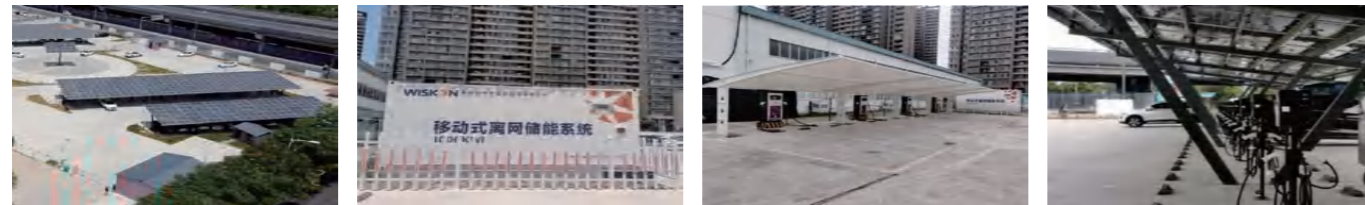
地面光伏电站 Ground Photovoltaic Power Station 1000KWh储能系统 1000KWh Energy Storage System 120KW直流充电桩 120KW DC Charging Pile 7KW交流充电桩 7KW AC Charging Pile
